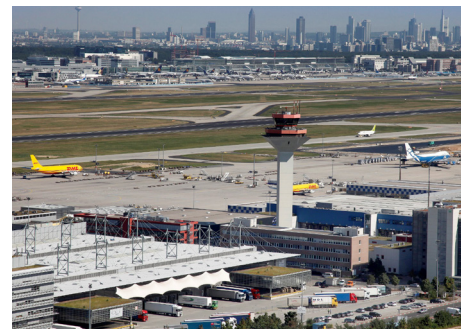
Cargo City South at Frankfurt Airport (Photo: Fraport AG/ Stefan Rebscher)
